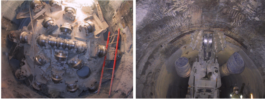
Figure 9.3: TBM Gripper type machine used for Neutrino tunnel at CERN (left) and road-header type machine (right).
