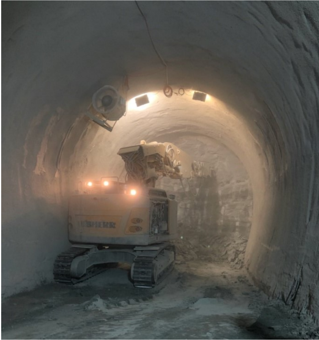
Figure 9.46: Rockbreaker used for cavern excavation at HL-LHC Point 1
