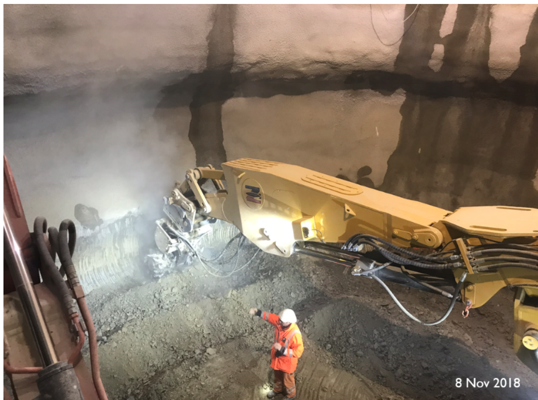
Figure 9.45: Excavator with hydraulic cutting heads being used at HL-LHC Point 1
