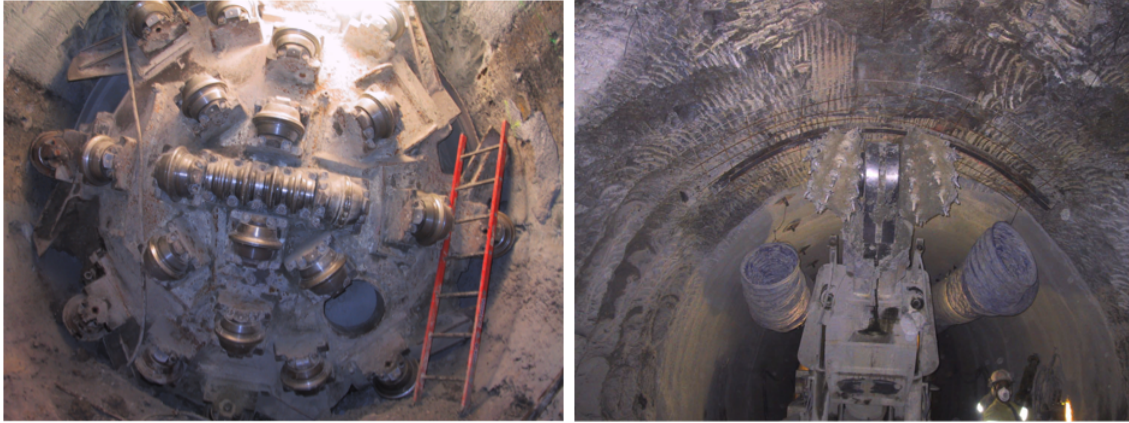
Figure 10.3: TBM Gripper type machine used for Neutrino tunnel at CERN (left) and roadheader type machine (right).
