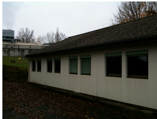
LHeC barack 561 in a protected area
