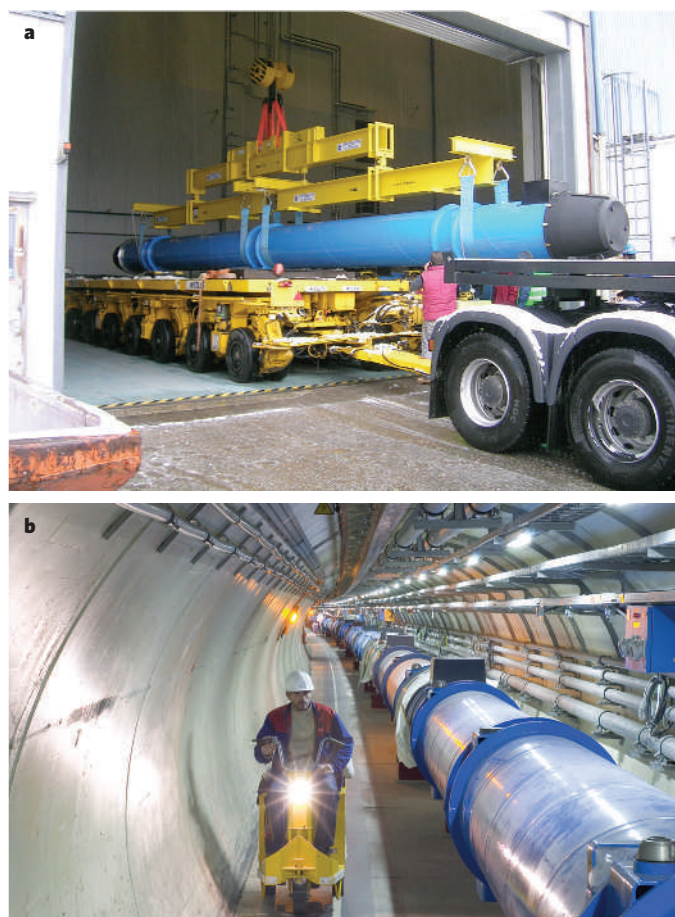
Figure 3 | Installing the LHC magnets. a, An LHC dipole ready for installation at the CERN site. b, Transport of LHC magnets in the tunnel, alongside installed elements, illustrating the tight space conditions for installation. Images reproduced with permission from CERN.
