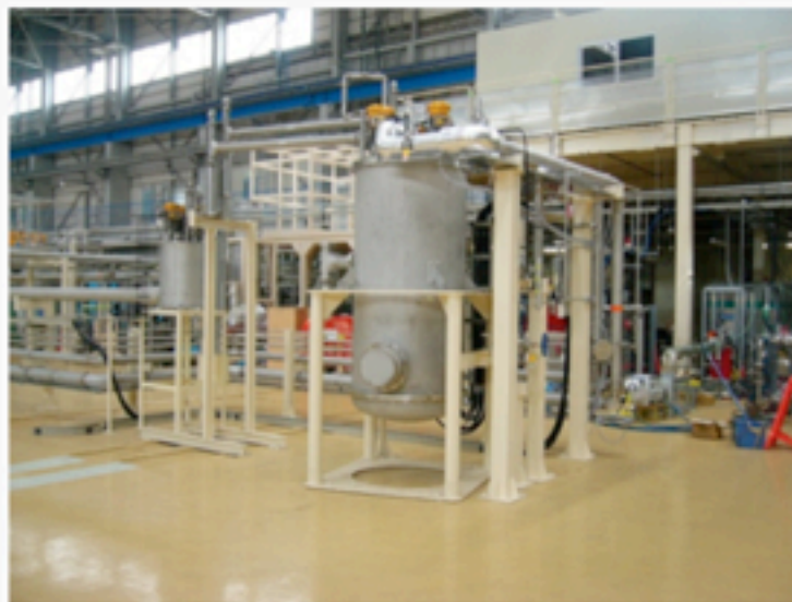
2K cold box and end box
