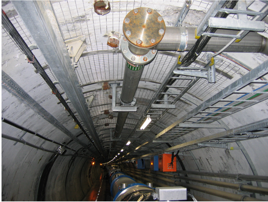
Figure 7.49: View of sector 4.
