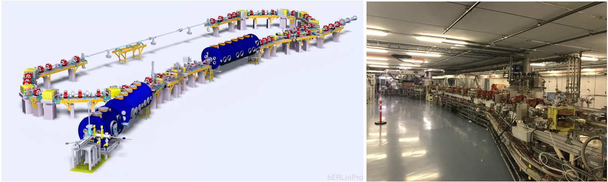
Fig. 6.2: Left: Structure of bERLinPRO, which is essentially complete apart from the 1.3 GHz linac module and the (upgraded) gun, the main hardware elements of the roadmap for bERLinPRO; Right: View from the dump position on the injector (at the back) and first racetrack part (June 2021).
