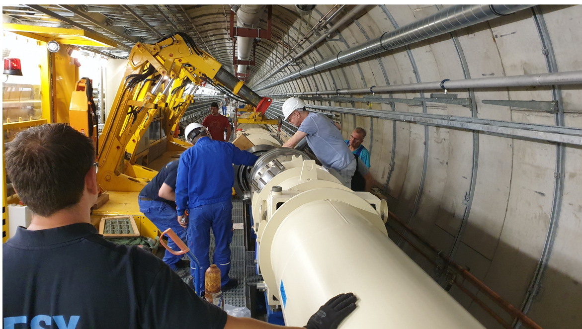
The ongoing installation of dipoles for ALPS II in the former HERA tunnel at DESY.
